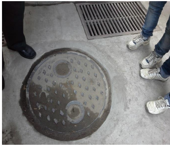
Storm Drain & Sewer Line Adjacent to each other
